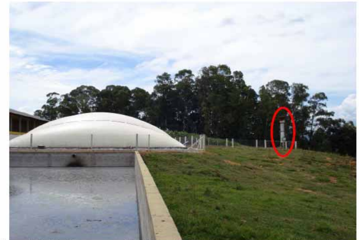
Figure A.4. – Biodigester system in white and enclosed flare system on the right in the farm of Sergio Tassi.
